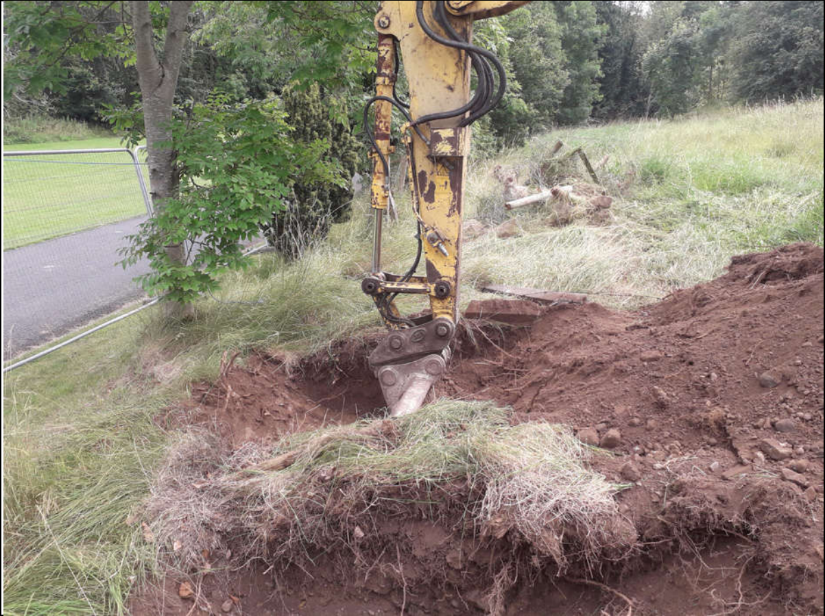
Plate 7: Slot trench under excavation, looking southeast
