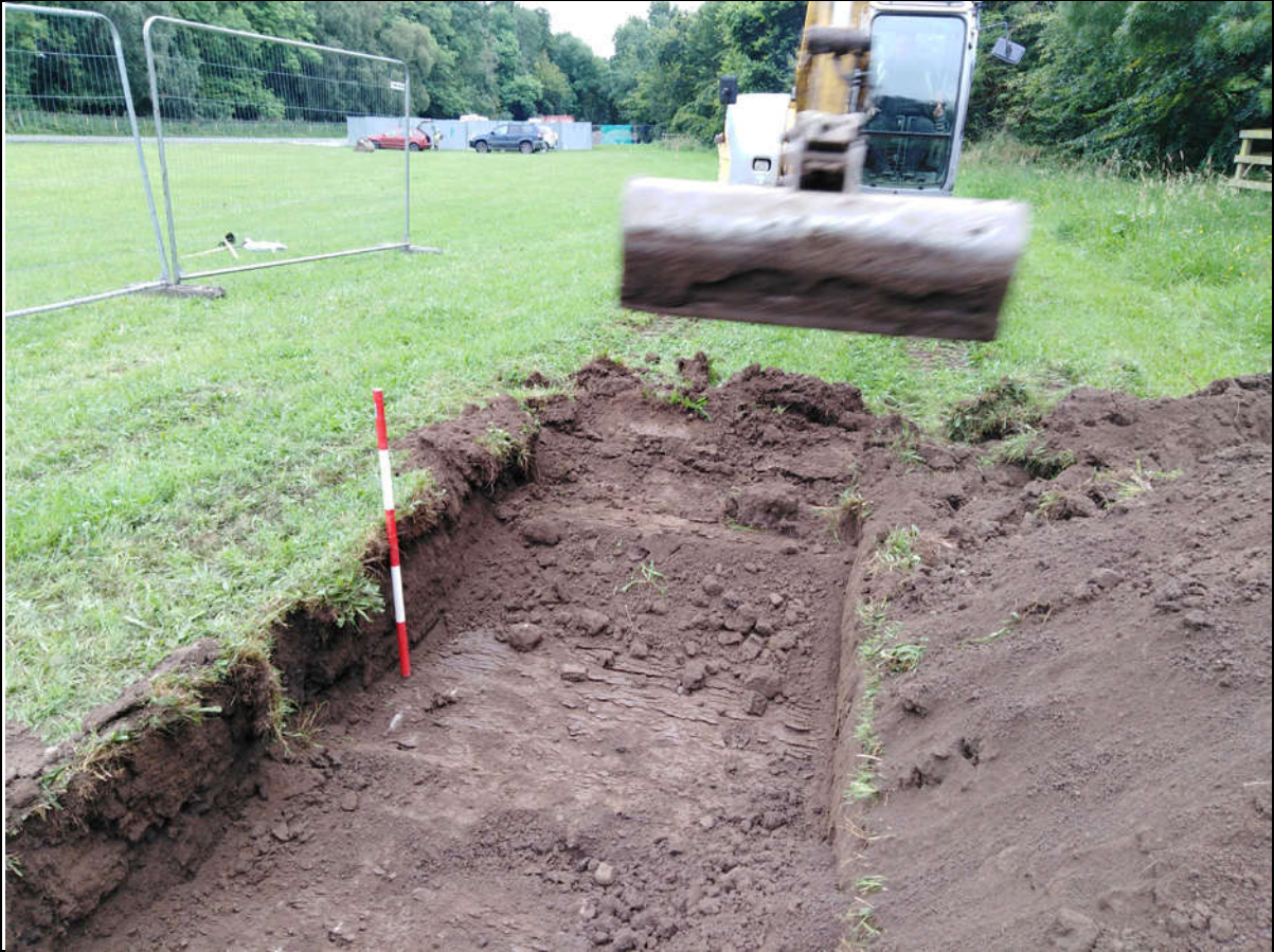
Plate 11: Trench 2.16 under excavation, looking southeast
