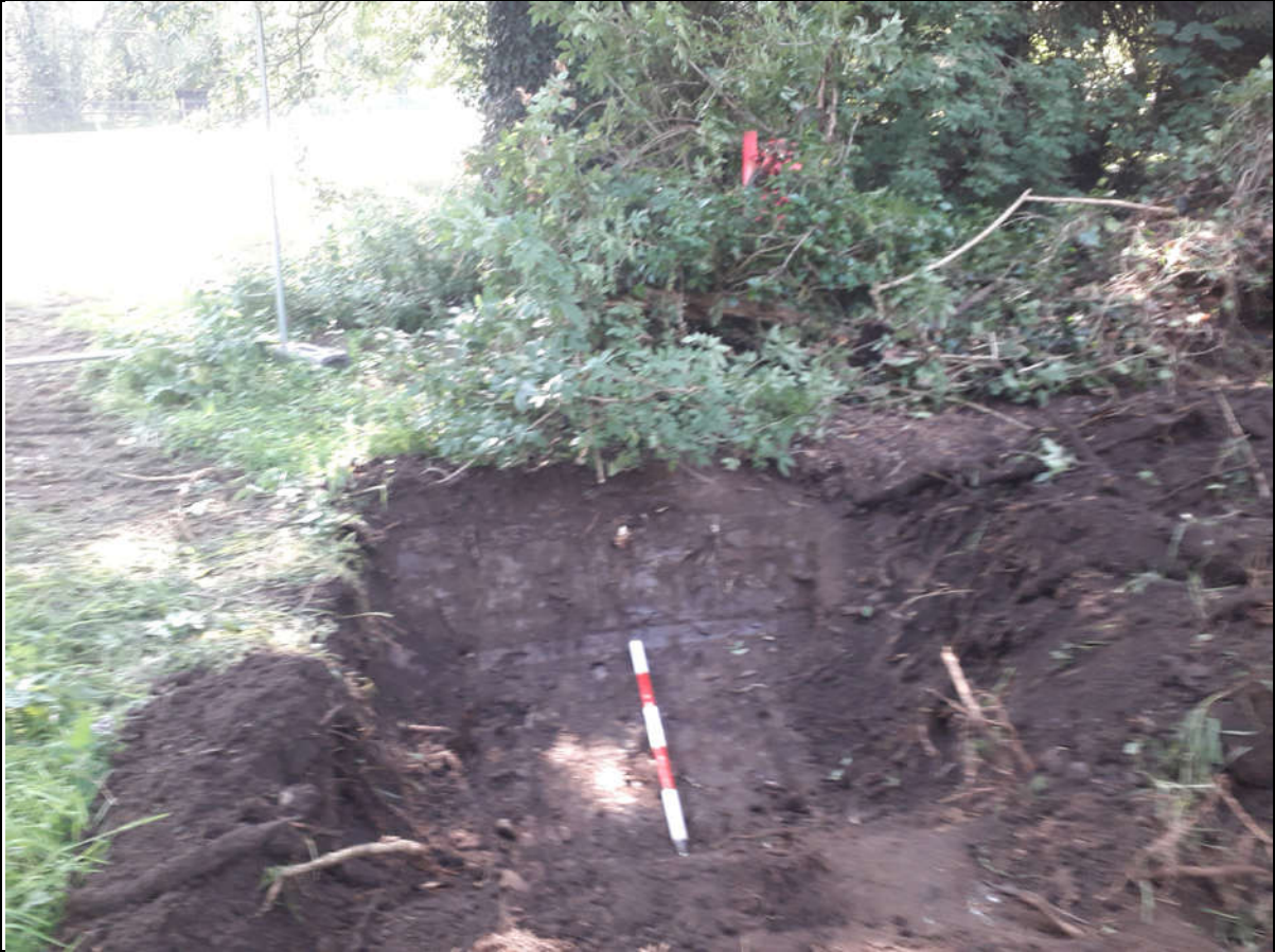
Plate 9: Slot trench close to Kerdiffstown Church, looking southeast
