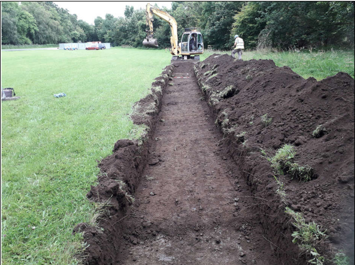
Plate 10: Trench 2.16, looking southeast
