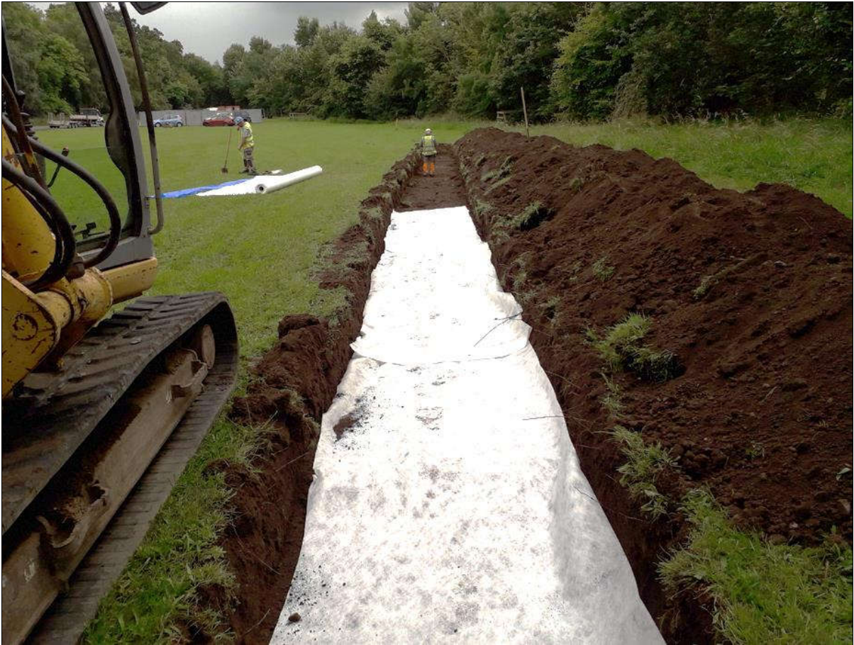
Plate 1: Terram lining base of Trench 2.16, Field Location 2, looking southeast
